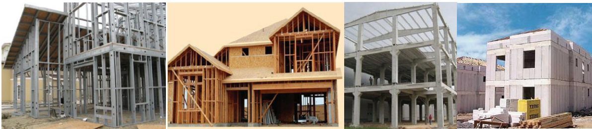
Figure 4. Cold formed steel frame, timber frame, reinforced concrete prefabricated and aerated concrete panel systems[Aksan, 2008] [Url-6] [Url-7] [Ytong, 2007].
